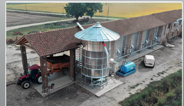
4 DRYERS PLANT + COOLING SILOS
